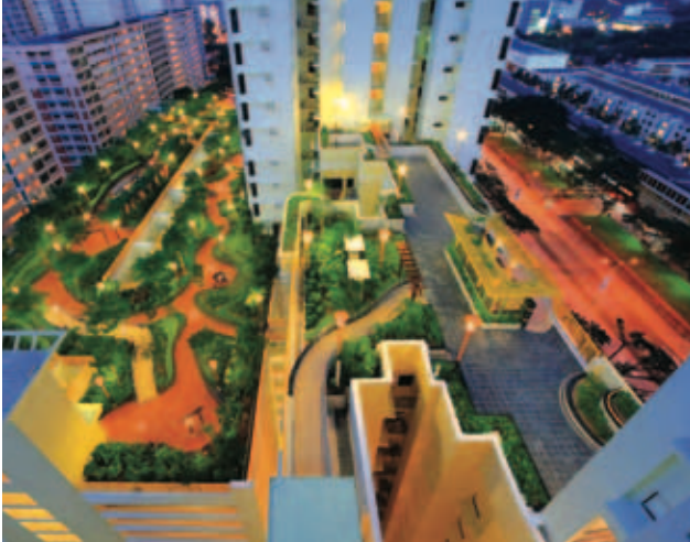
Central Horizon, which took second prize in the Built Category of the SIA-NParks Skyrise Greenery Awards, renews the sense of communal living by creating generous rooftop landscaped gardens. These are joined to and independently accessible from each apartment block in the precinct.
