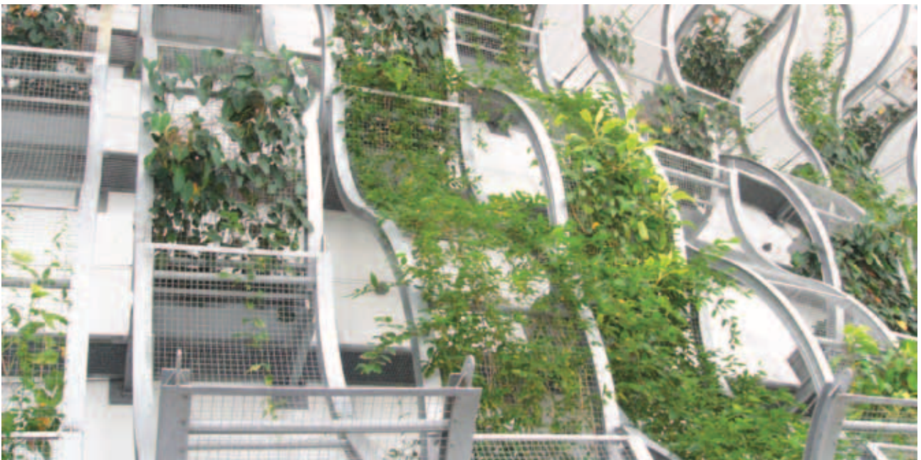
Besides their aesthetic benefits, green walls – such as this one in Fusionopolis – also help to cool their surroundings, cleanse the air of dust particles, and provide additional habitats for urban biodiversity. They can also optimise land use in high-rise environments, and boost the value of properties.
